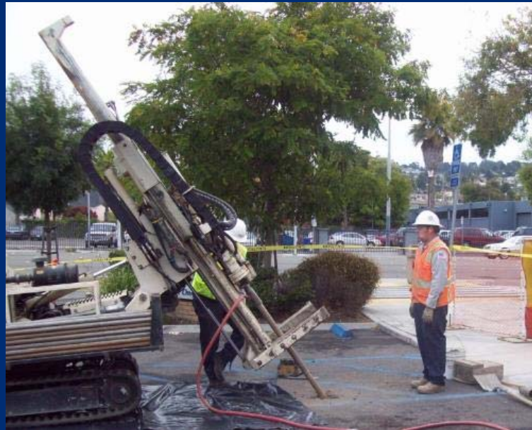
Direct-push injection of 10% by weight gypsum slurry (angled implementation possible, but not planned for this site)
